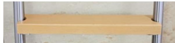
Holzstufe an Rundrohr, Wooden step mounted at circular tube,
